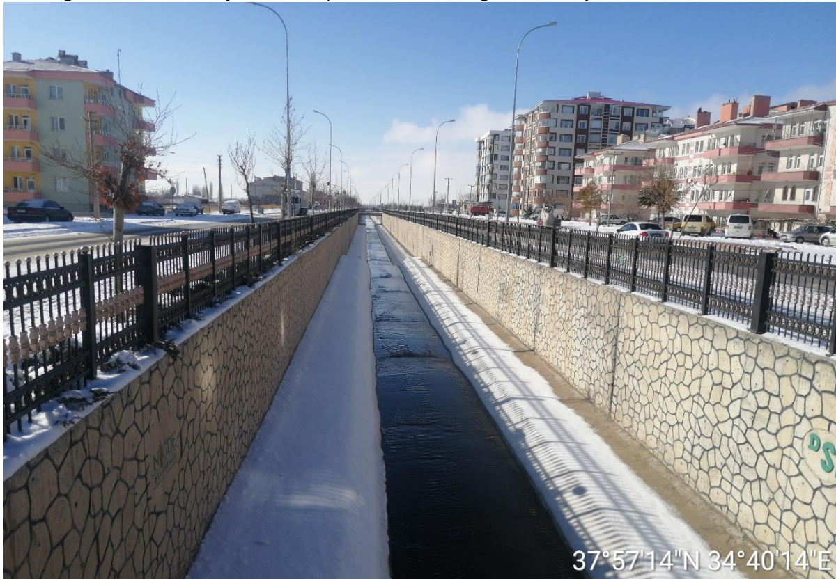
Figure III.4 Kizilca Stream, where the discharge of the rainwater network is planned
